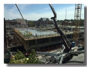
Concrete mixing trucks constantly alternate loading the massive pumper as the 2nd floor is being poured (1010/16). Over 25,000 square feet of concrete per floor. That's over 10x the average home size built last year.
